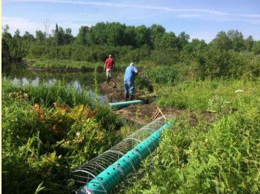
Five years ago, to control the water level from a large beaver dam that resulted in a trail closure, our club purchased a Clemson Leveler (see photo). Developed by Clemson University and field tested by the Minnesota DNR, it changes water flow so that beavers cannot sense it and as a result don't attempt to plug the leveler. Our source in Minnesota for the Clemson Leveler no longer builds them. I decided to create a more robust design, and make them available to ATV clubs.
